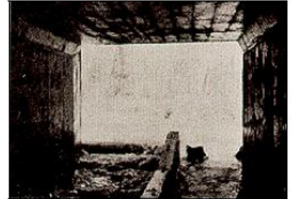
Figure VI-7--Fish Baffles in Culvert
