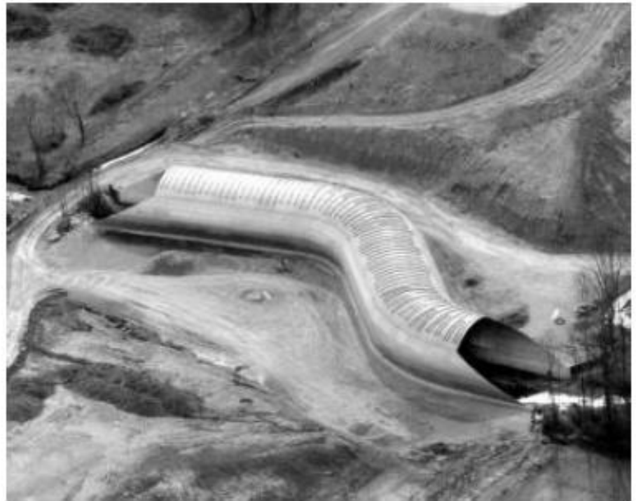
Figure VI-4--Culvert with a Horizontal Bend (Contech)
