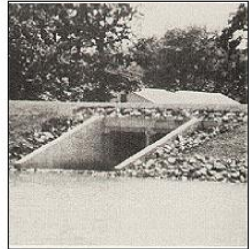
Figure VI-1--Stormwater Management Pond with Culvert as Outflow Control Device
